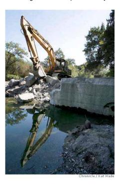
A backhoe removes parts of the Sunol Dam on Alameda Creek, a project to help steelhead spawn. Chronicle photo by Kat Wade
